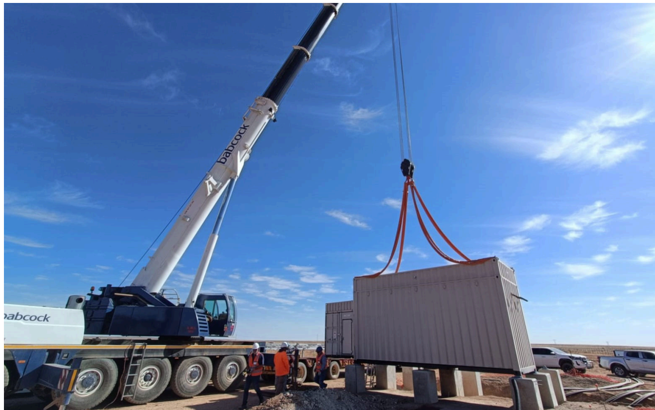
CONTAINERISED SUBSTATION AND BATTERY ENERGY STORAGE ON BOLTABLE TWISTLOCK FOUNDATIONS
