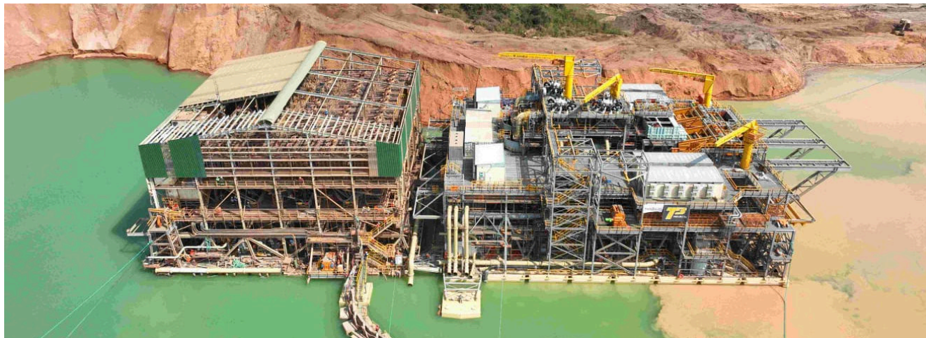
THE WET CONCENTRATOR PLANT AFLOAT IN ITS MINING POND, MOMA
